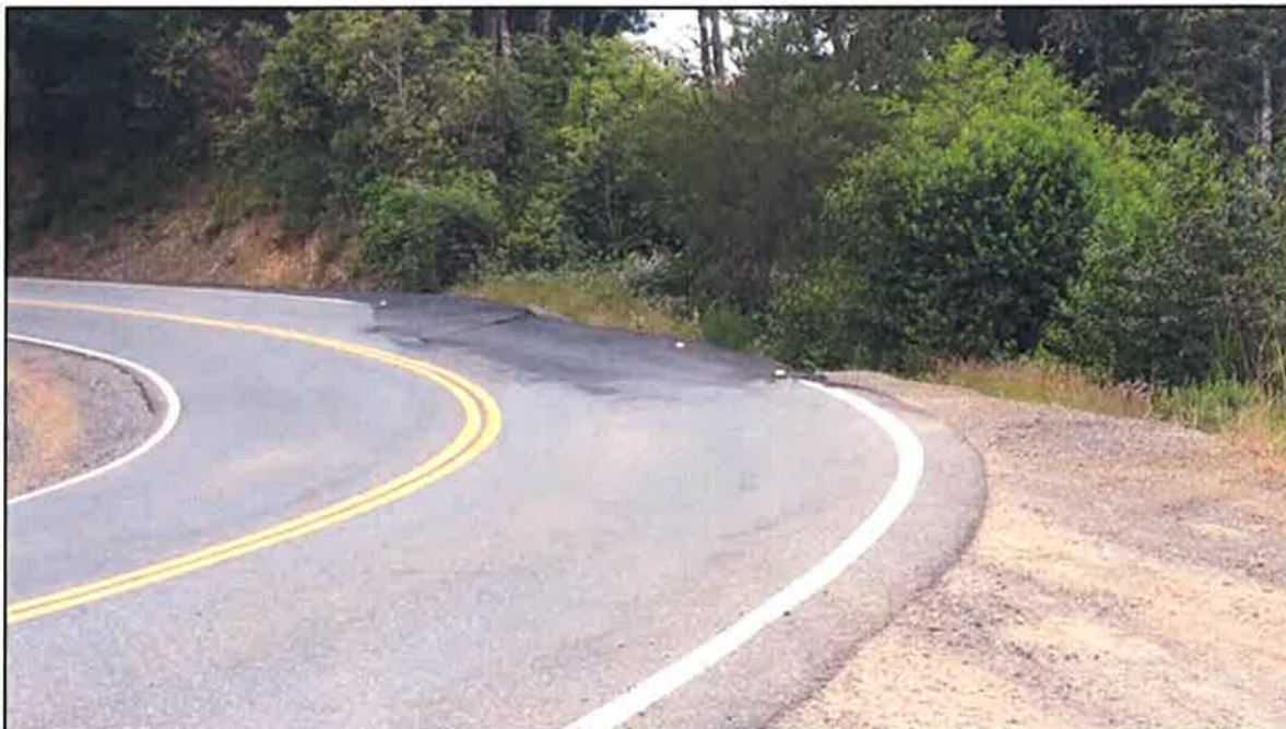
Looking northwesterly at a view of the paved access road, where the road has subsided and needs to be repaired.
