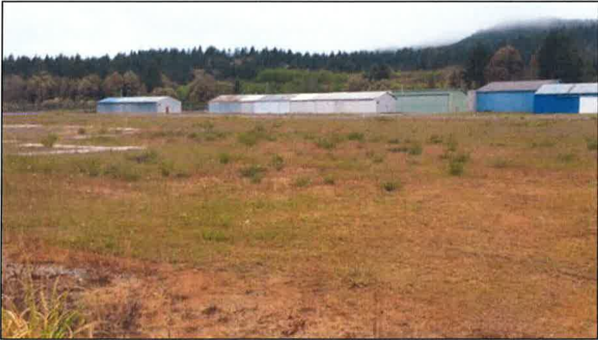
Looking northeasterly across the airfield at a view of airplane hangers on the subject site from near the west gate.
