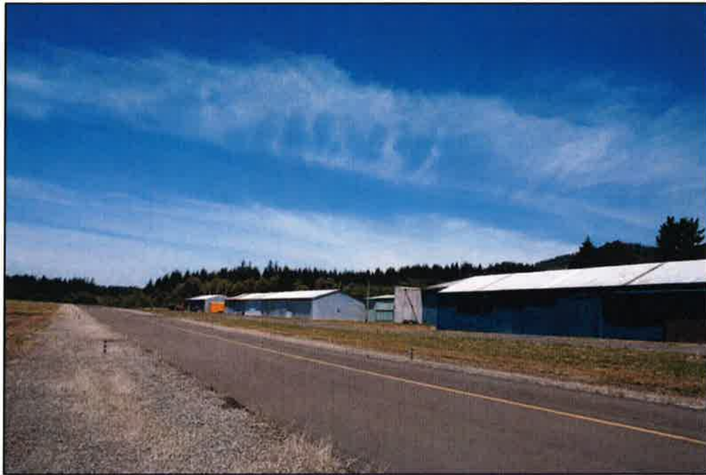
Looking northerly at a view of a runway and hangars. These improvements are owned by leasehold ownerships paying monthly fees for the land area that they sit on.
