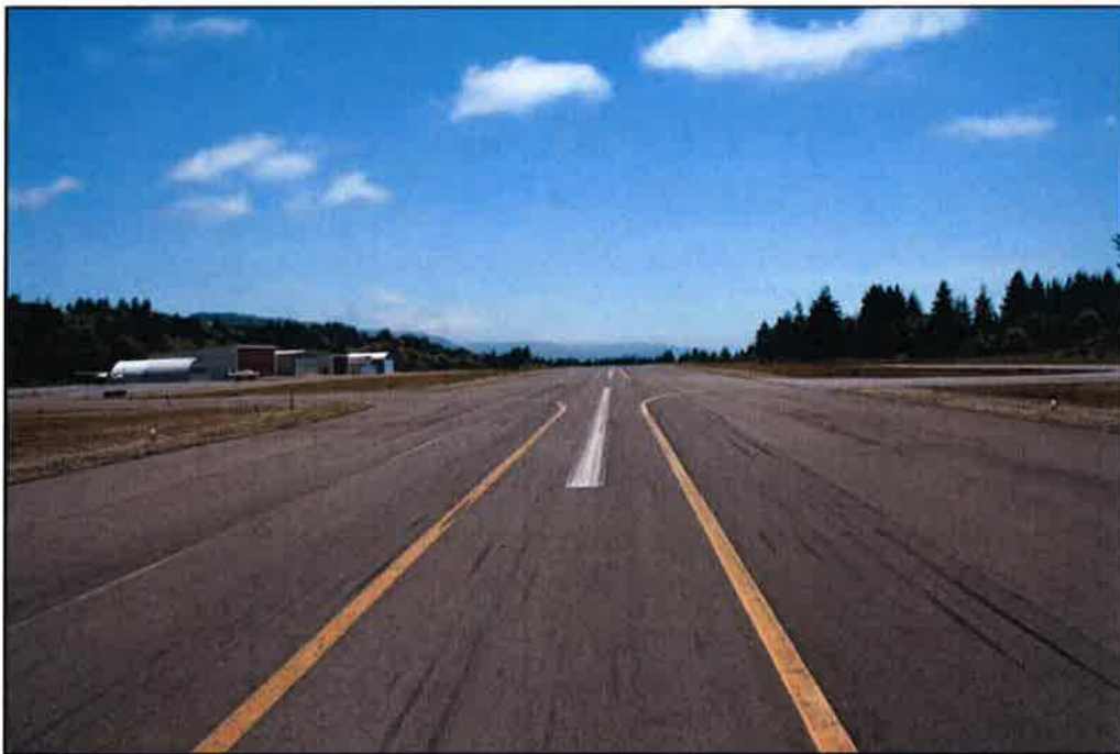
Looking southerly at a view of a runway and hangars.
