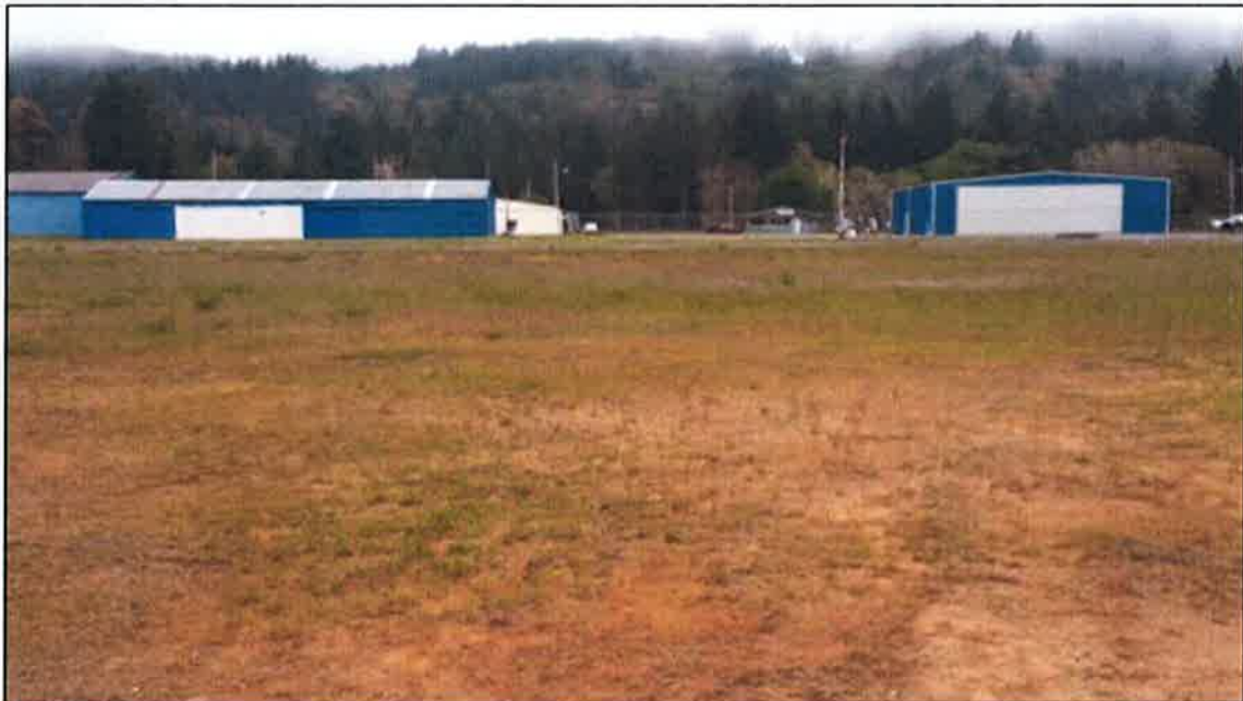
Looking easterly across the airfield at a view of airplane hangers on the subject site from near the west gate.
