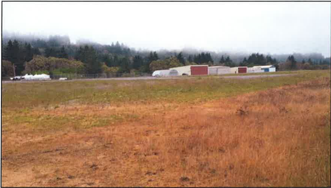
Looking southeasterly across the airfield at a view of airplane hangers on the subject site from near the west gate.
